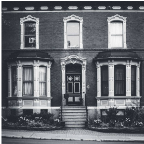
A classic Bed-Stuy brownstone facade, restored stoop and window surrounds intact.
